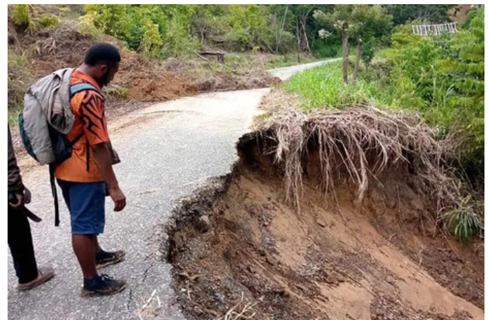
The aftermath of landslides in PNG in March 2024 (Al Jazeera, 2024).
